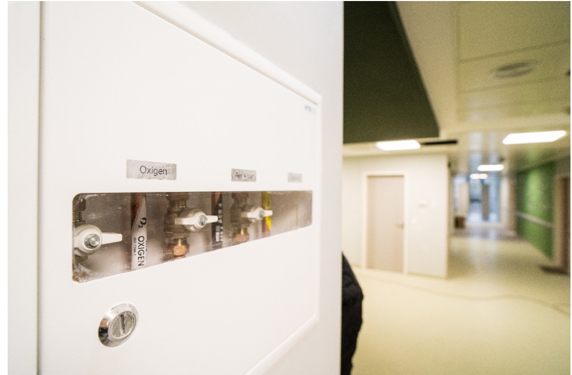
Medical gases switchboard
