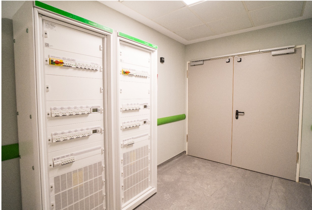
Electric and IT switchboard
